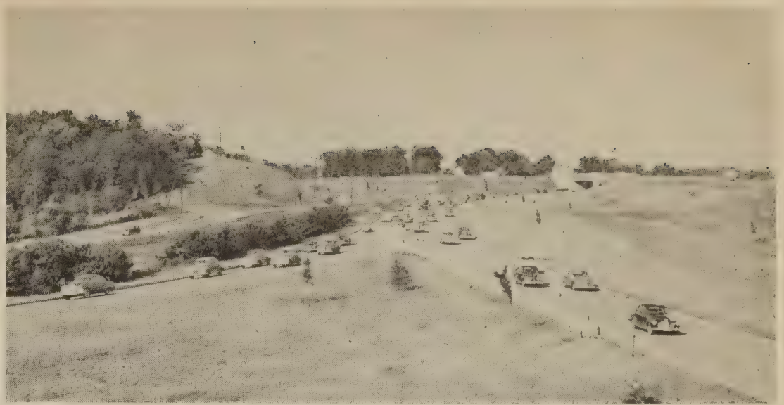
Weaving section for north-bound traffic at the junction of Shirley Highway and Washington Boulevard, Arlington, Va.
